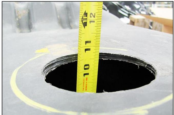
5. Measure the depth from the highest surface around the drilled hole to the highest surface of the tank floor.
